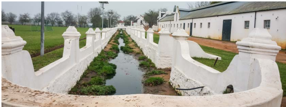
Baroque-walled drainage channel at Elsenburg
