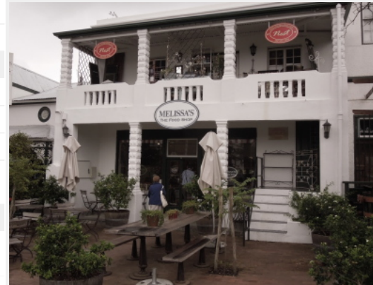
DATE OF PHOTOGRAPH(S): DECEMBER 2013
