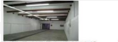
Figure 6: View of the end of the 19 th century addition, facing eastwards.
